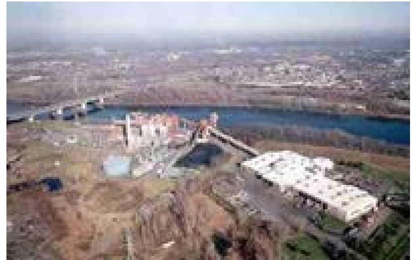
Hartford trash-to-energy plant
